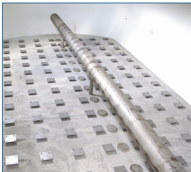
A horizontal filter with the underdrain installed (internal view).
